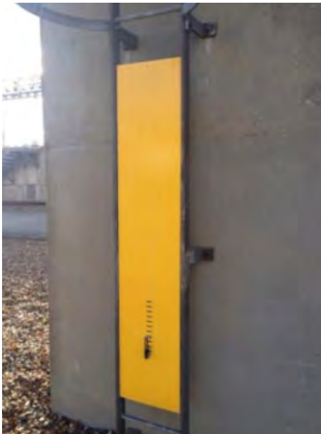
> Ladder Guard Installed
